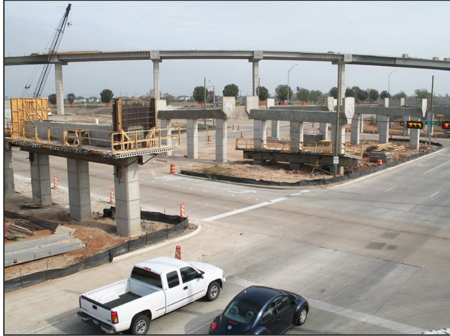
West Park Tollway
